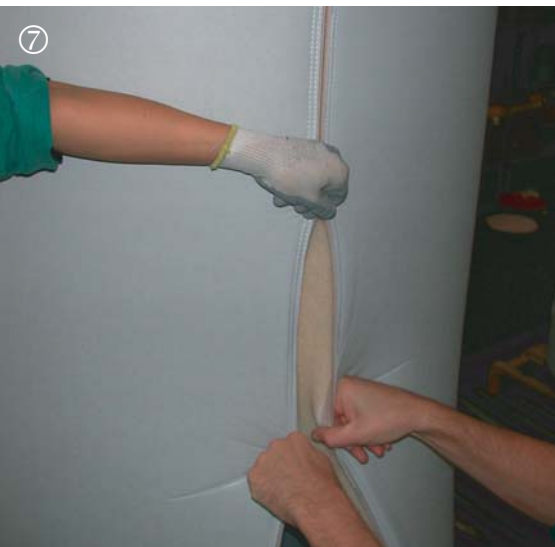
Pictures showing how to mount soft-foam insulation with a PVC sheet on a storage water heater.
