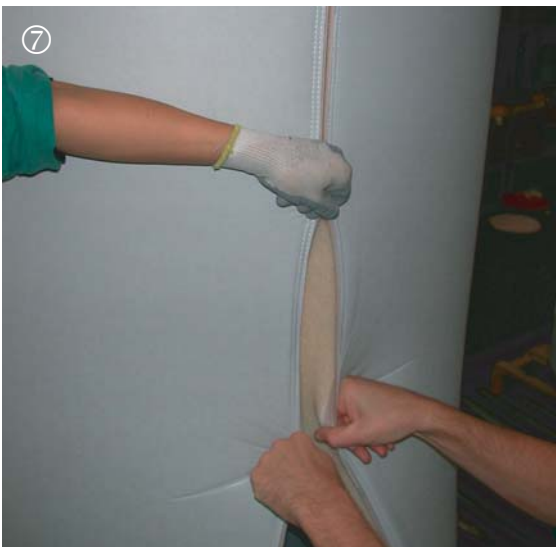
Pictures showing how to mount PVC coated flexible foam insulation on a storage tank.
