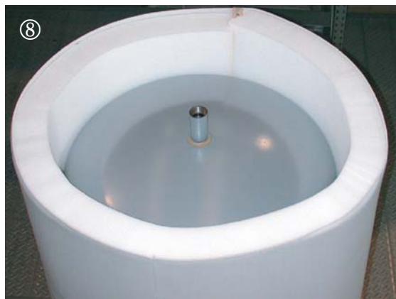
Pictures showing how to mount PVC coated flexible foam insulation on a storage tank.
