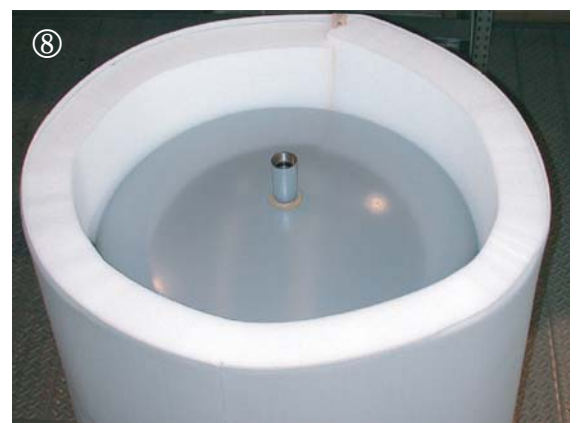
Pictures showing how to mount soft-foam insulation with a PVC sheet on a storage water heater.
